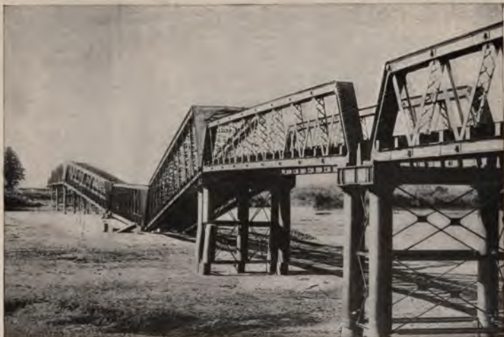
A. NAGARAGAWA BRIDGE AFTER THE MINO-OWARI EARTHQUAKE IN JAPAN ON OCTOBER 28, 1891. (After Kikuchi.)
